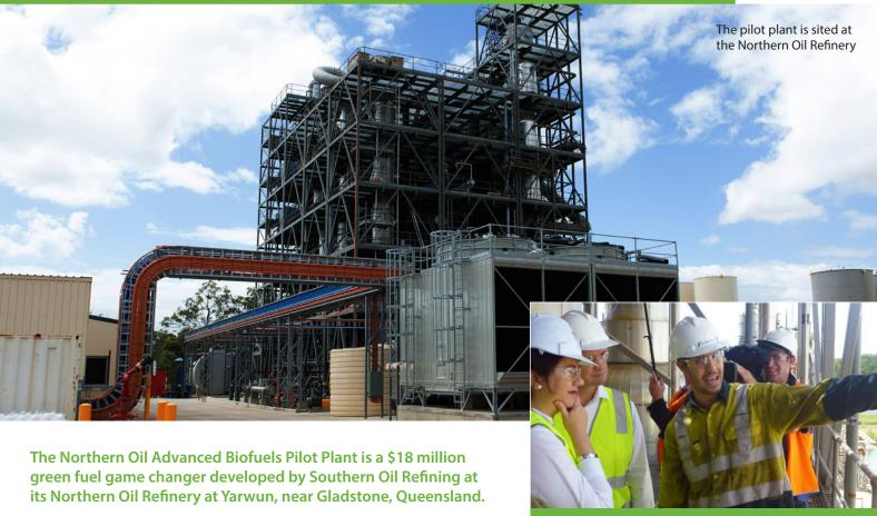
The pilot plant will use biomass and waste material such as sugarcane bagasse and prickly acacia as feedstock for the production of biocrude oil, which will be refined into saleable kerosene and diesel products.
